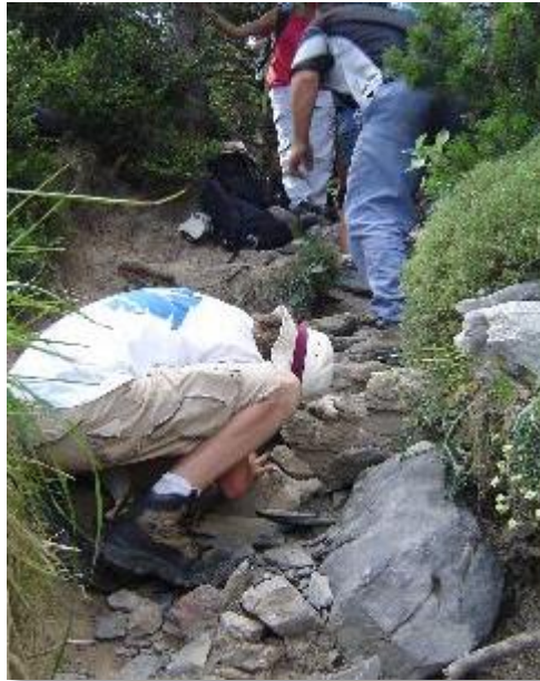
Photo 21. Work to restore a path in a protected area.
